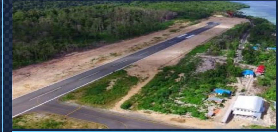
Maratua Island Domestic Airport Operational
