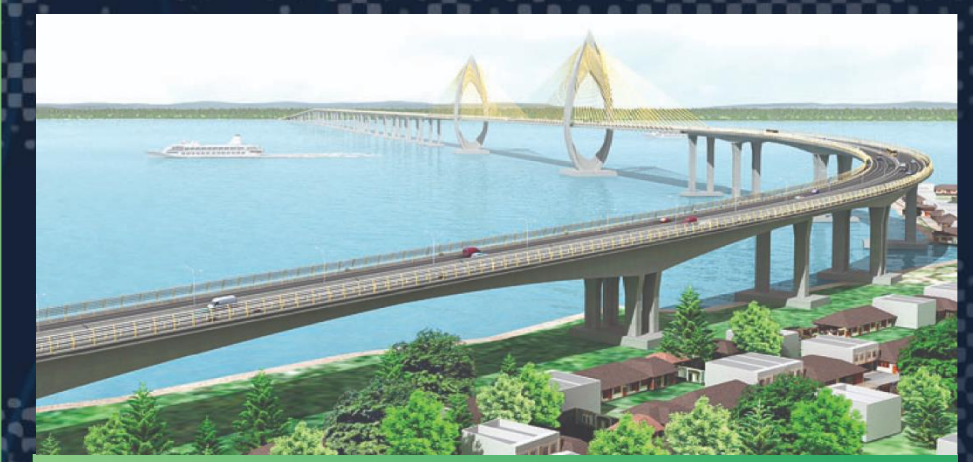
Toll Bridge - Balikpapan Bay Offered for Investment
